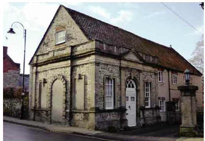
Figure 3. The Old Pump House at Glastonbury as it is today, with classical façades superimposed on existing cottages.
